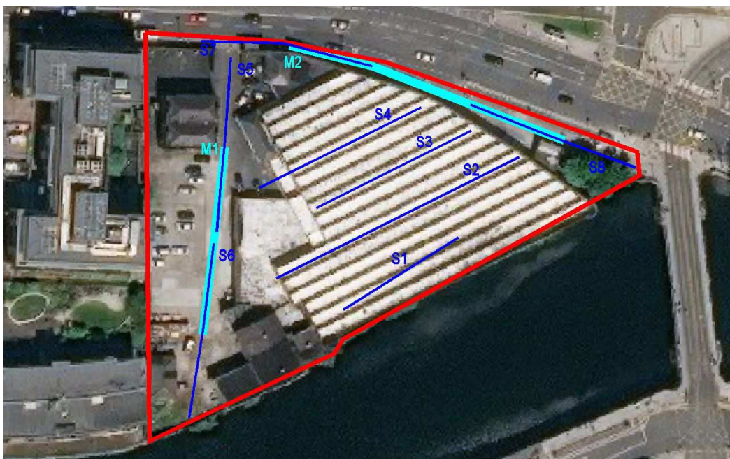
Fig 3.1: Aerial photo (site outlined in red).
